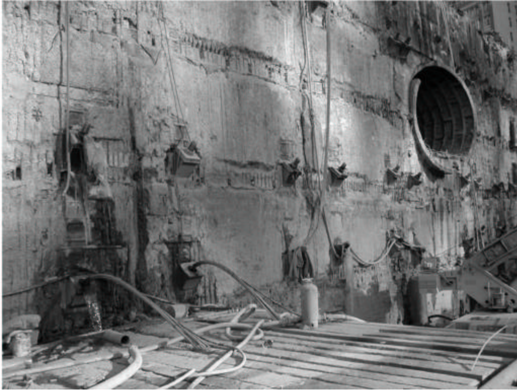
Two rows of Anchors, PATH tunnel
