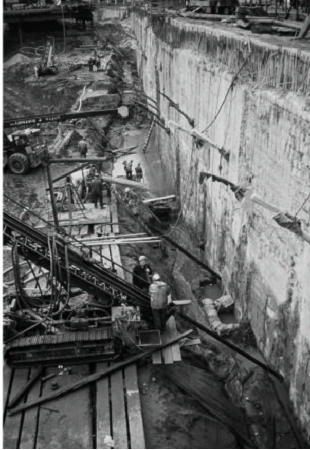
Wall Anchor Installation
