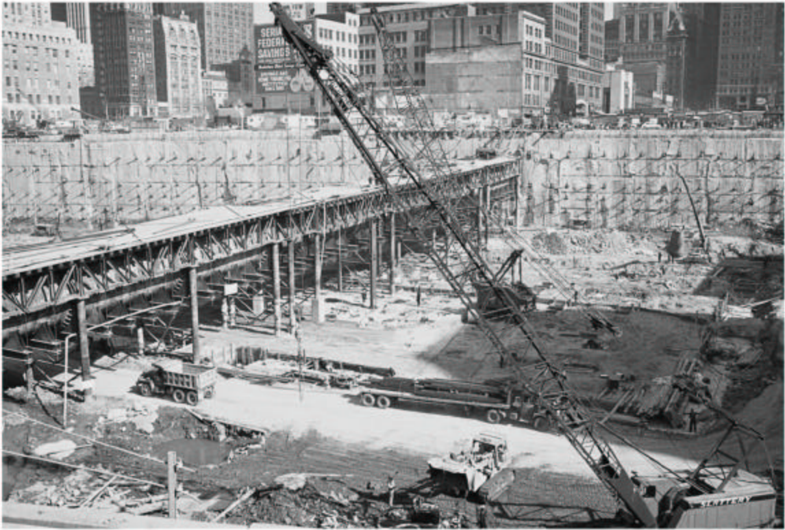
Completed Greenwich Slurry Wall & supported PATH Tube
