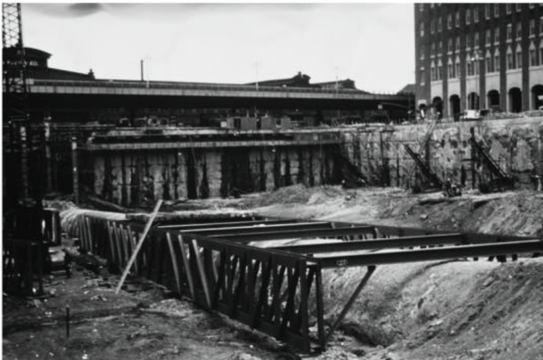
Truss Supporting North PATH Tube, berm, anchor installation
