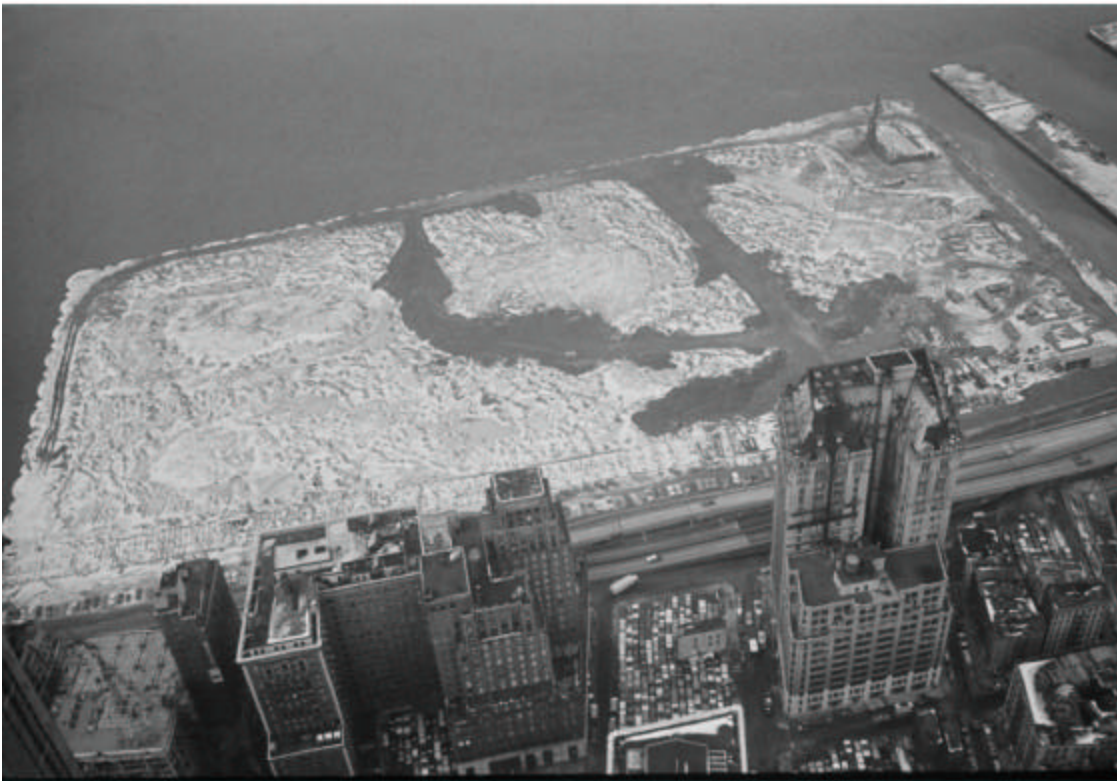
Land Fill site (essentially completed, installing Pump Station sheeting)
