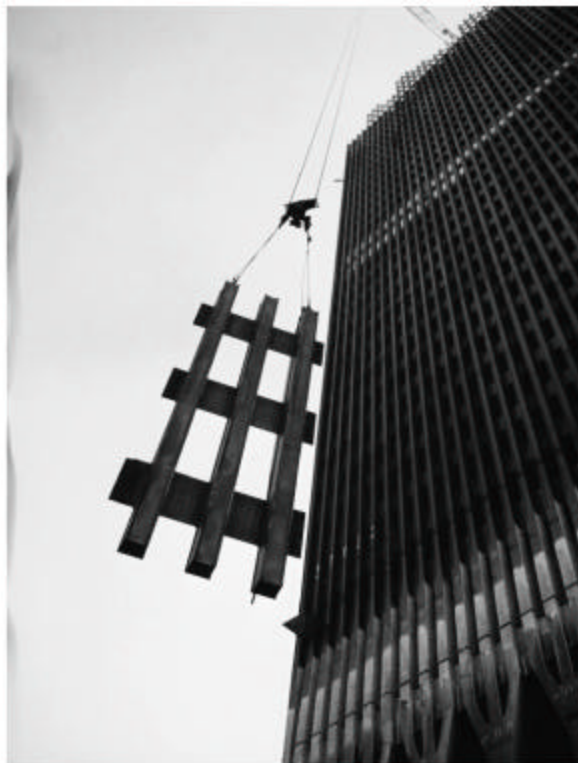
Lifting prefabricated outside wall section
