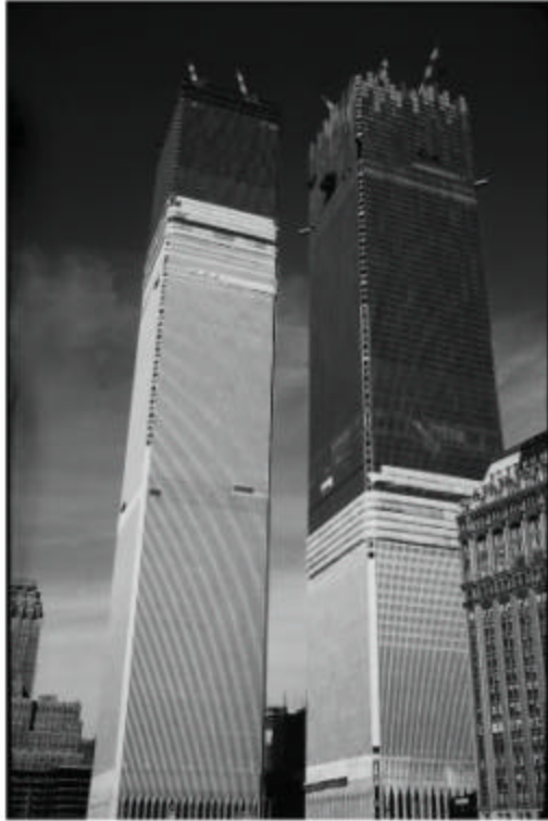
Towers construction observed from basement
