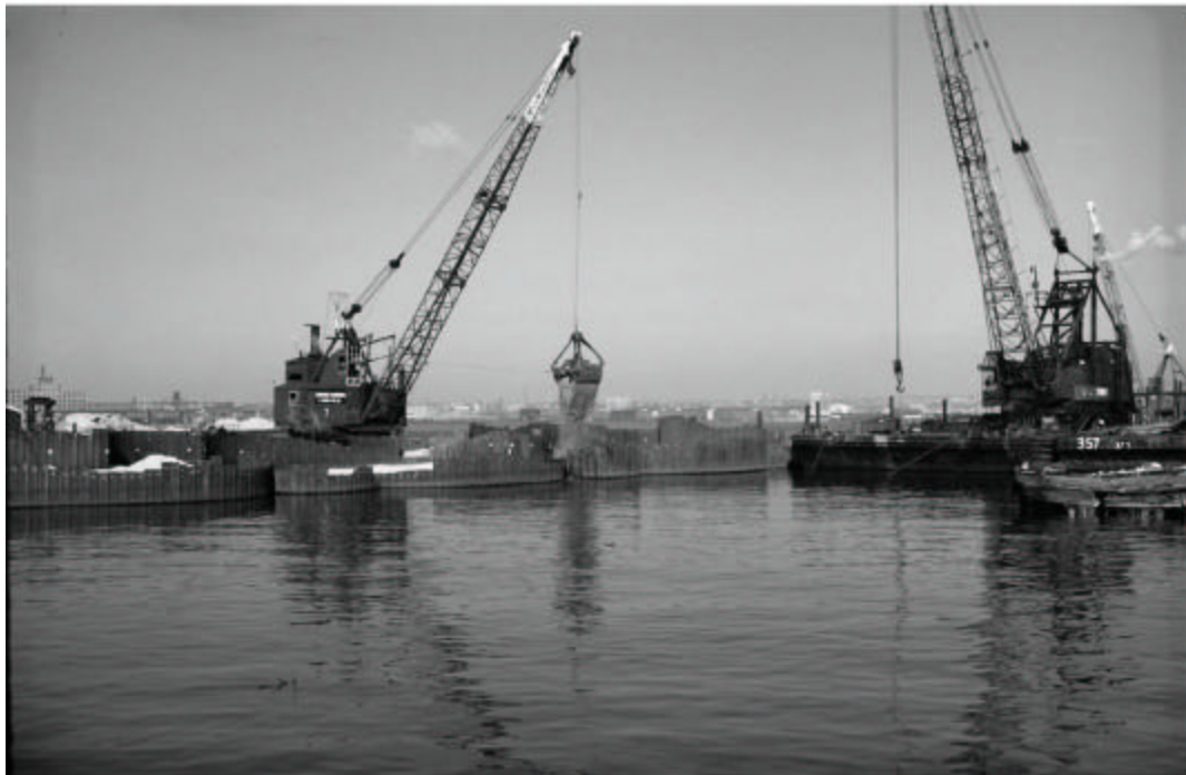
Cofferdam Construction (Cofferdam being filled with Sand)
