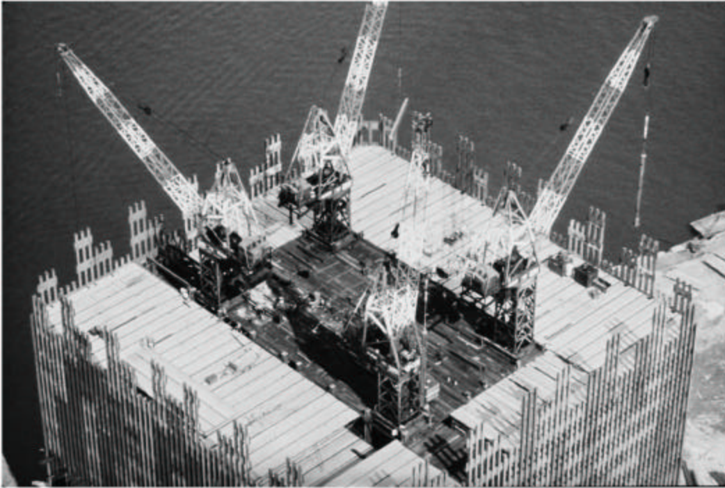
Steel erection utilizing Kangaroo cranes
