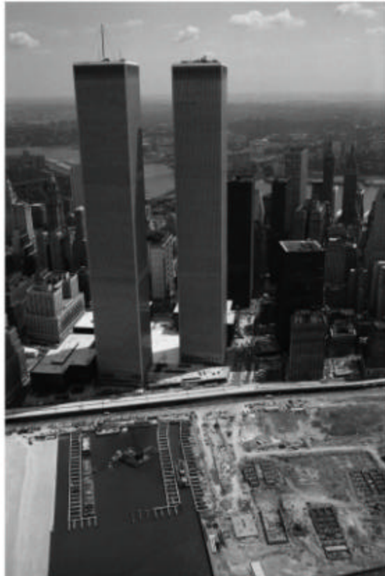
Towers completed, Battery Park construction
