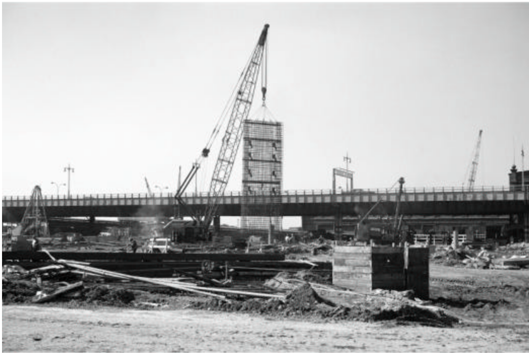
Slurry Wall Reinforcing Cage being lowered
