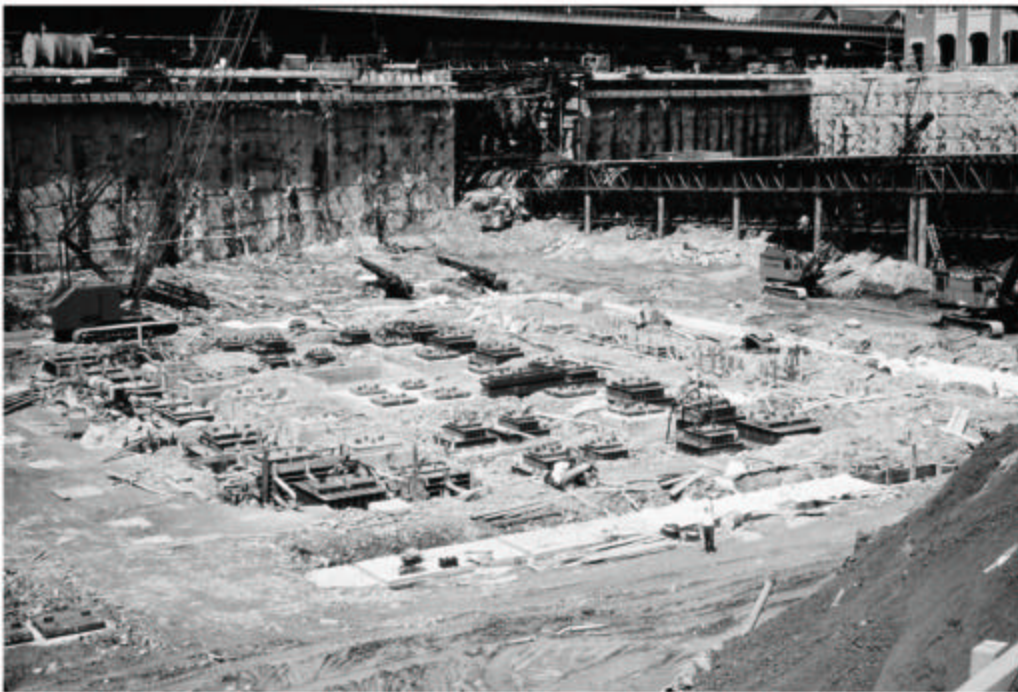
Tower Footing Construction, PATH Tube structurally supported
