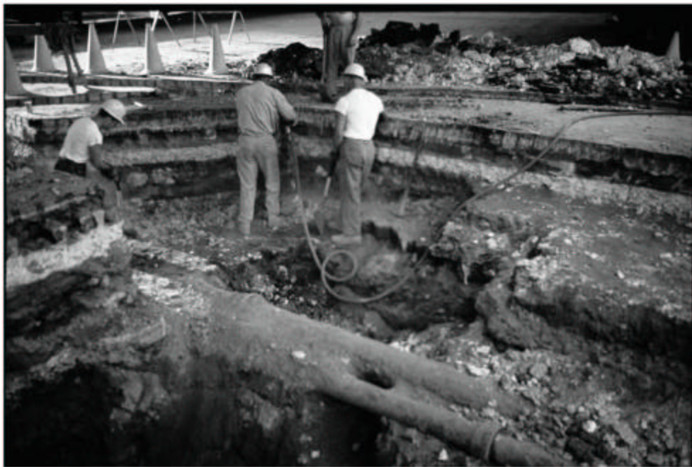
Pre- Construction Utility Excavation
