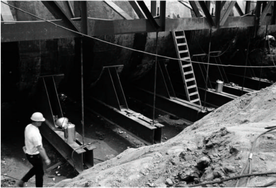
Caisson Supporting PATH truss
