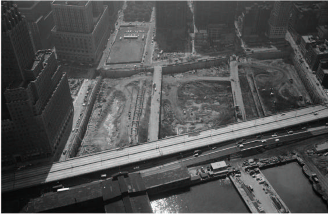
Basement excavation, construction bridges, north PATH tube, AT&T building
