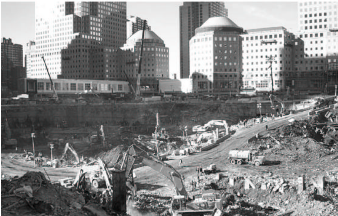
Wall & Excav Equip, Demol. Looking at Winter Garden, Earth Ramp
