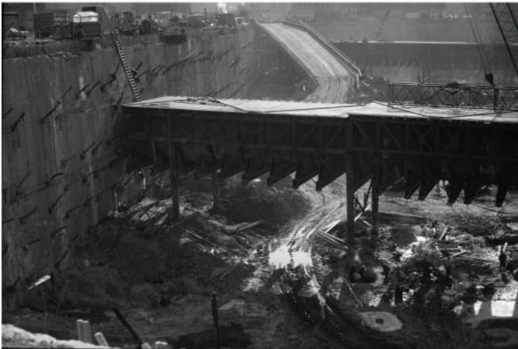
Supported PATH Tube at Greenwich Street Slurry Wall, beneath BMT Subway
