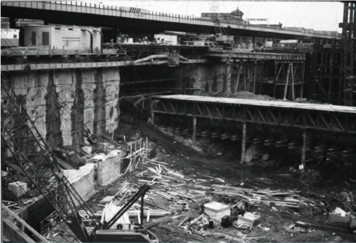
Supported PATH tube at West Street Slurry Wall
