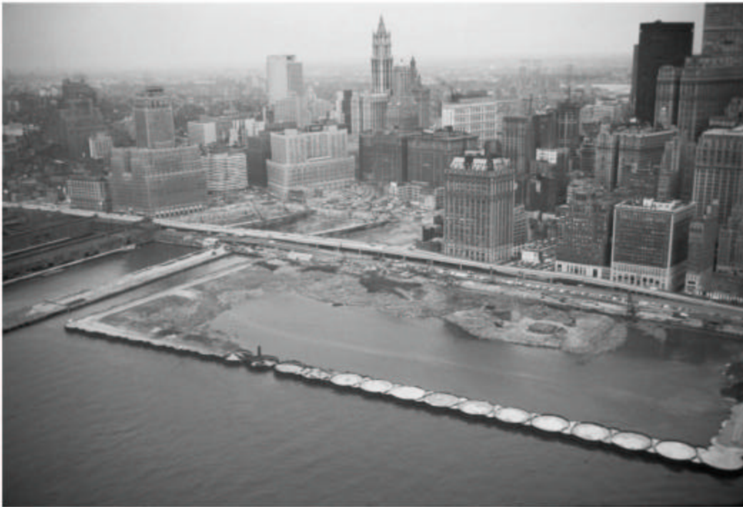
Site of future Battery Park City (Cofferdams mostly completed, filling with WTC materials started)
