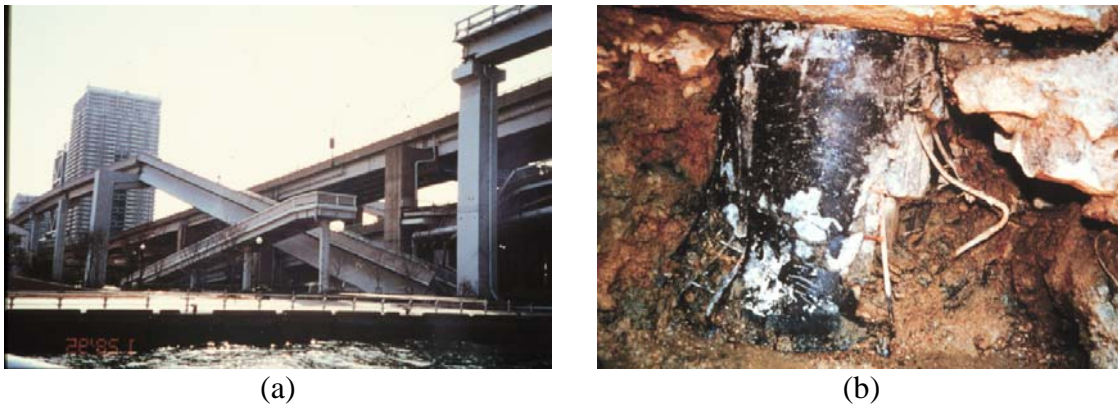
Figure 1. Damage caused by lateral spreading to piles during 1995 Kobe earthquake in Japan: (a) railroad bridge (M. Kumura, Kyoto U.); and (b) damage to reinforced concrete pile foundation (K. Tokimatsu, Tokyo Inst. of Technology).
