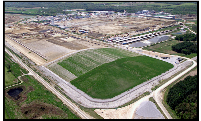
Figure 5. Aerial photo of OSDF in 2002 with various cells being constructed, operated, and closed.
