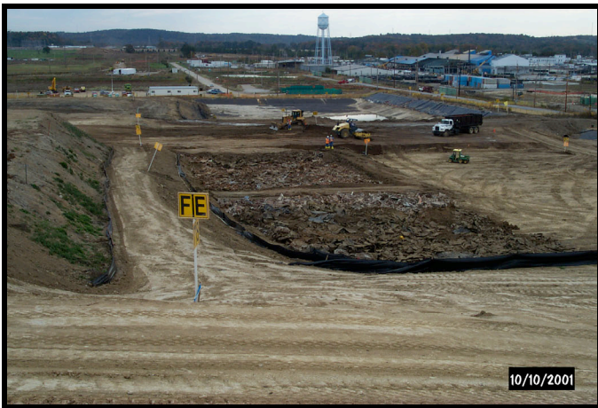
Figure 9. Typical grid system for placement of impacted material, with Category 2 material being placed in the center of the photograph. Placards were used to identify the grids to facilitate placement and construction documentation. Cell stormwater catchment area is also visible in upper-center portion of photograph.
